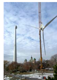
Turbine erection at Exhibition Place in Toronto. Courtesy of WindShare
